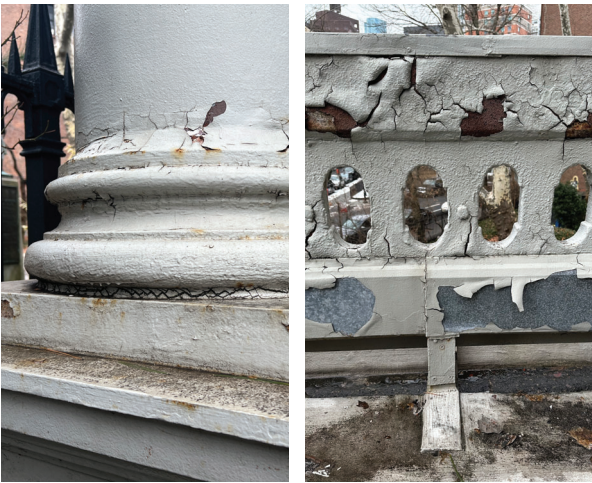
A12-1 - REPAIR CAST IRON PORTICO
