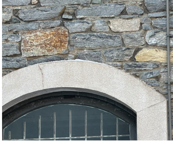
A11-1 - REPAIR STONE & WINDOW SURROUNDS
