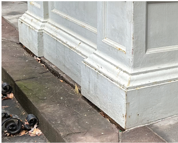
A17-2 - RESET DISPLACED CURBS AT PORTICO
