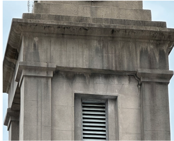
A31 - CLEAN MASONRY FACADES
