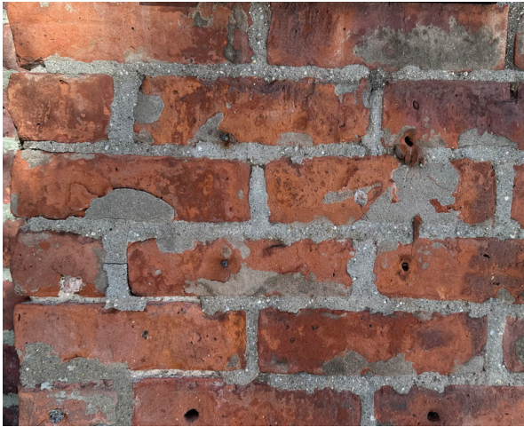
A30 - REPOINT PARISH HALL MORTAR JOINTS
