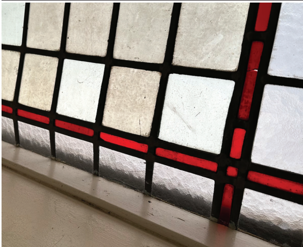
A33 - REPAIR STAINED GLASS WINDOWS
