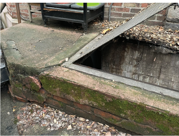
A17-1 - REPLACE AREAWAY VAULT DOORS AND CURB
