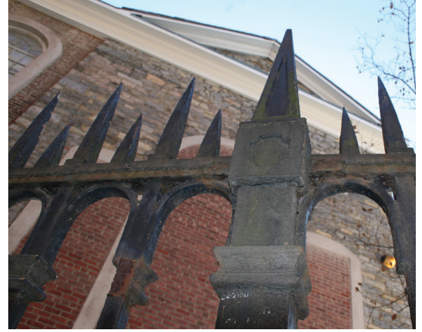
A20 - REFINISH METAL PORTION OF SITE FENCE
