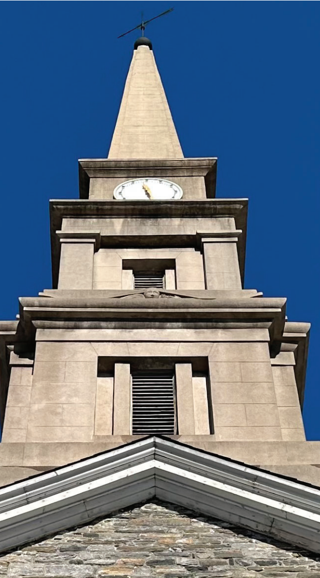
Stucco generally sound and in good condition from the ground.
