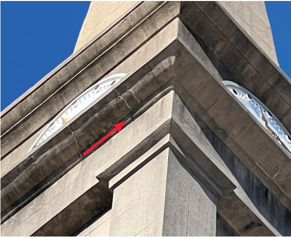
A11-3 - REPAIR BELL TOWER STUCCO
