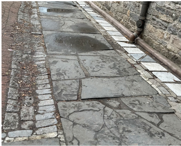
A53 - REPAIR SITE PAVING TO PARISH HALL
